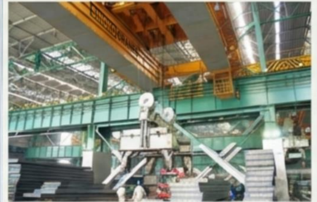
Billet Handling Crane
